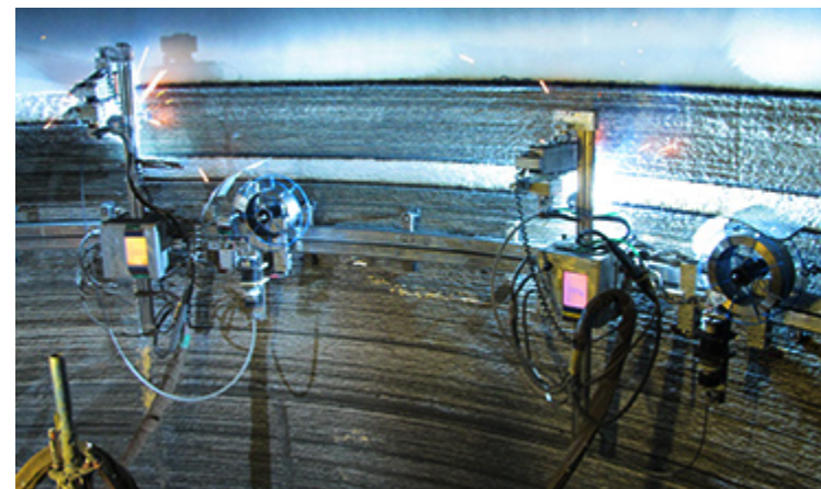
Coke Drum Repair
